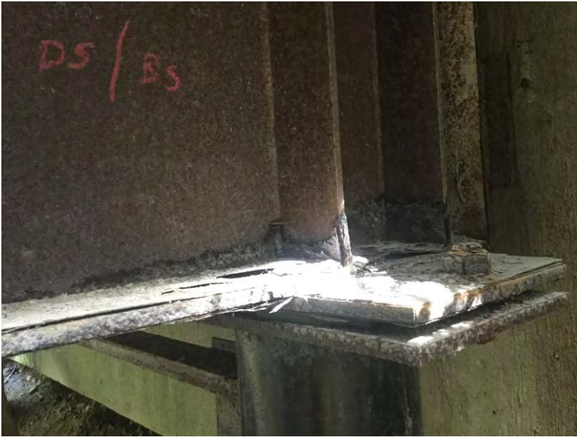
Left Bank Abutment when facing downstream
