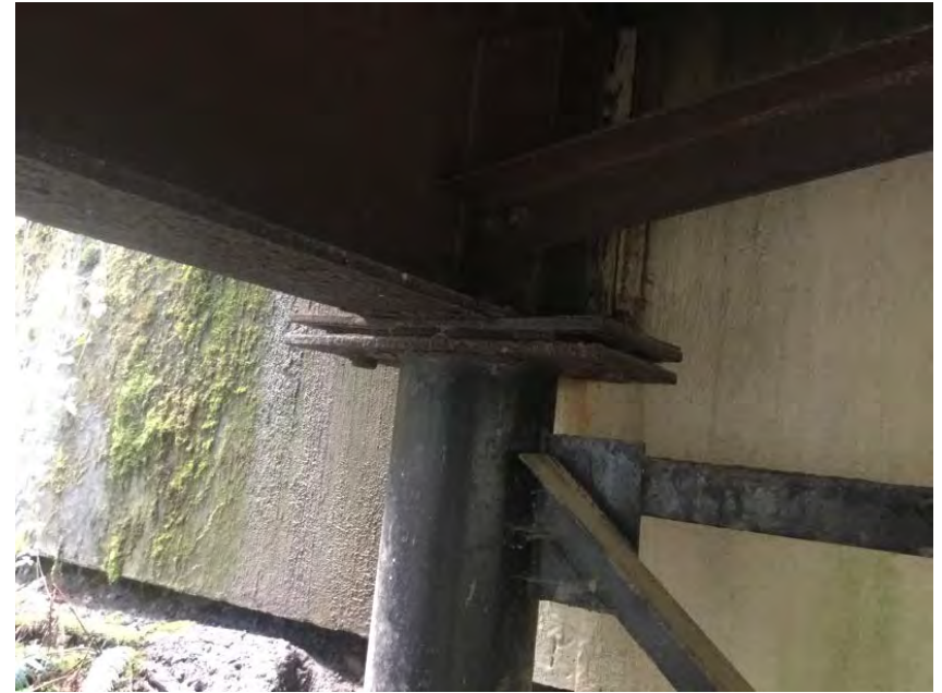
Right Bank Abutment when facing downstream - DS side
