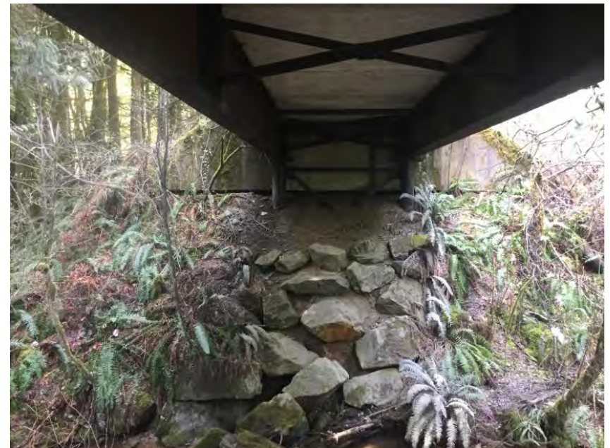
Right Bank Abutment when facing downstream
