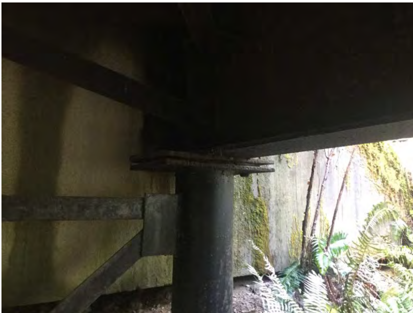
Right Bank Abutment when facing downstream - US side
