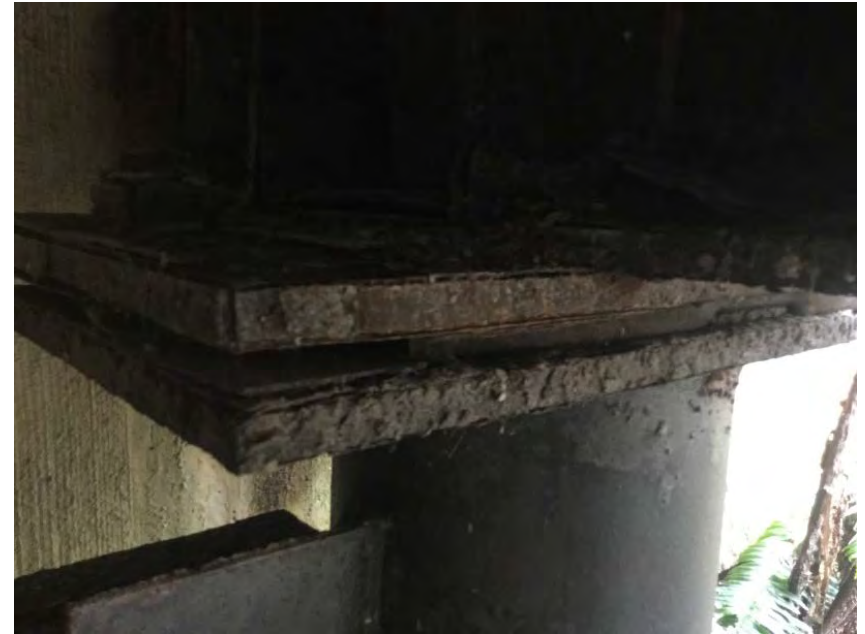
Right Bank Abutment when facing downstream
