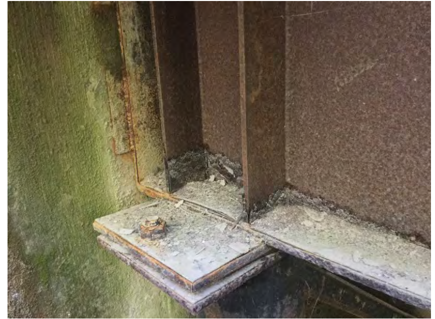
Left Bank Abutment when facing downstream - left abutment upstream side
